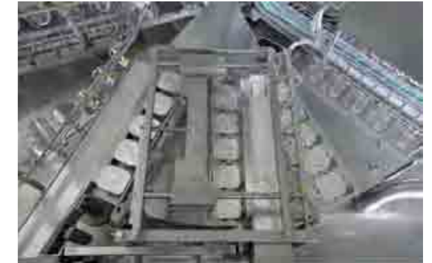
Ejection of the finished package onto good lanes (for final packaging) or bad lanes with cross-checking. If a package is determined to be bad, it is checked if it arrives on the "bad lane" and that it is definitely missing from the "good lane".
