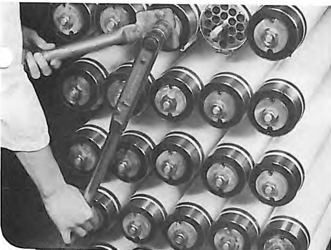
11. Tighten end caps to correct torque using 2-pin tool to prevent rotation of module. Correct tightening torque is 20lb. ft. (2.8 kg.m) for pressures up to 40 kg/cm 2 and 60lb. ft. (8.3 kg.m) for pressures up to 80 kg/cm 2 .
