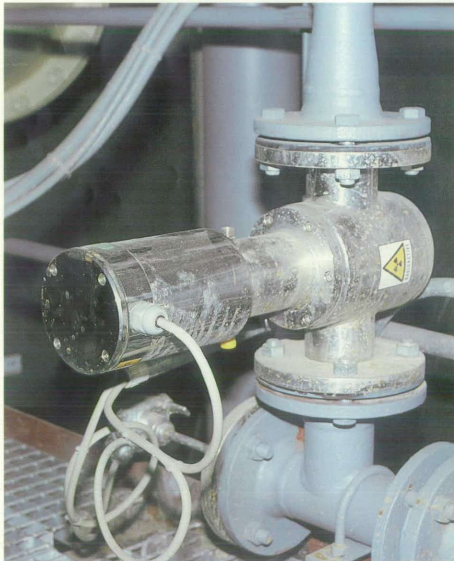
Density measurement in a flue gas desulfurizing facility.
